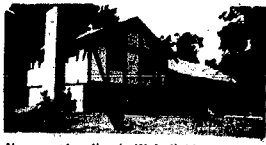
New construction in Wakefield.
